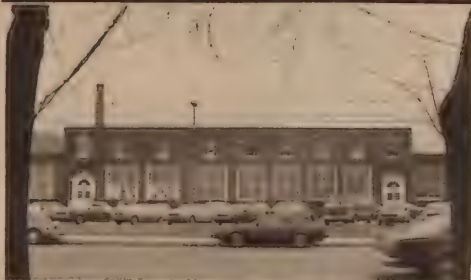
The Administration Building as it looks from across West Third Street. The building is slated to be torn down within the next 60 days. [Photo by Richard E. Kopp, Jr.]
